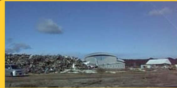
The gym and much trash in ruin by Tsunami in Ishinomaki
